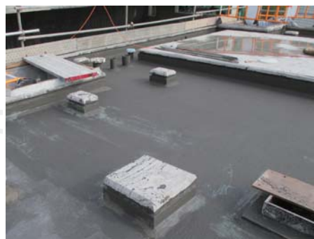
Water penetration of other market-available waterproofing coatings.
